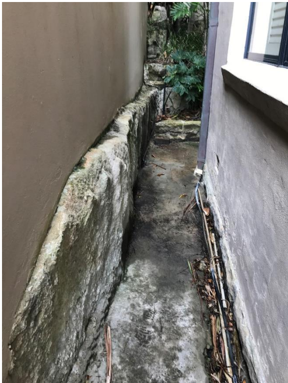
Photograph 5: Sandstone excavation along east boundary, middle portion
