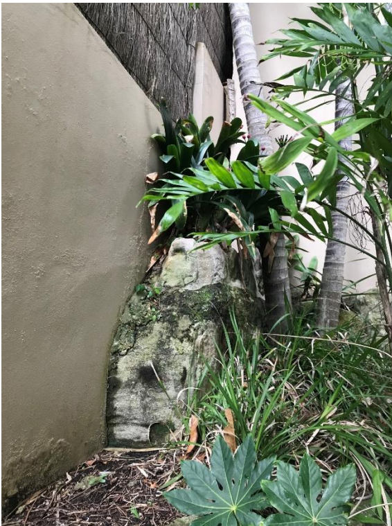
Photograph 4: Sandstone excavation along east boundary, south portion
