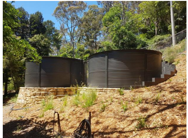
Existing water tanks, rear of site
