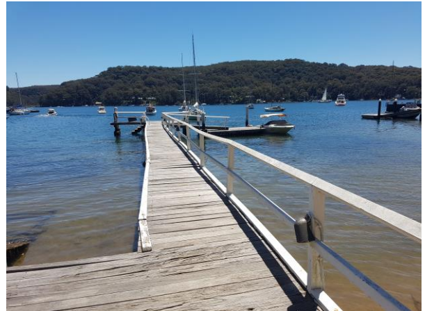
Existing jetty and deck, looking NW
