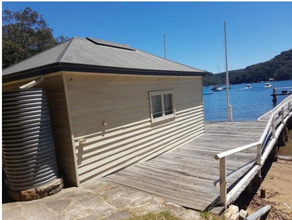
Existing boat shed, looking NW
