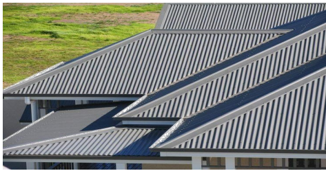
MT-01 COLOURBOND METAL ROOF SHEETING POWDERCOAT FINISH 'IRONSTONE' OR SIMILAR WHERE MARKED ON ELEVATION.
