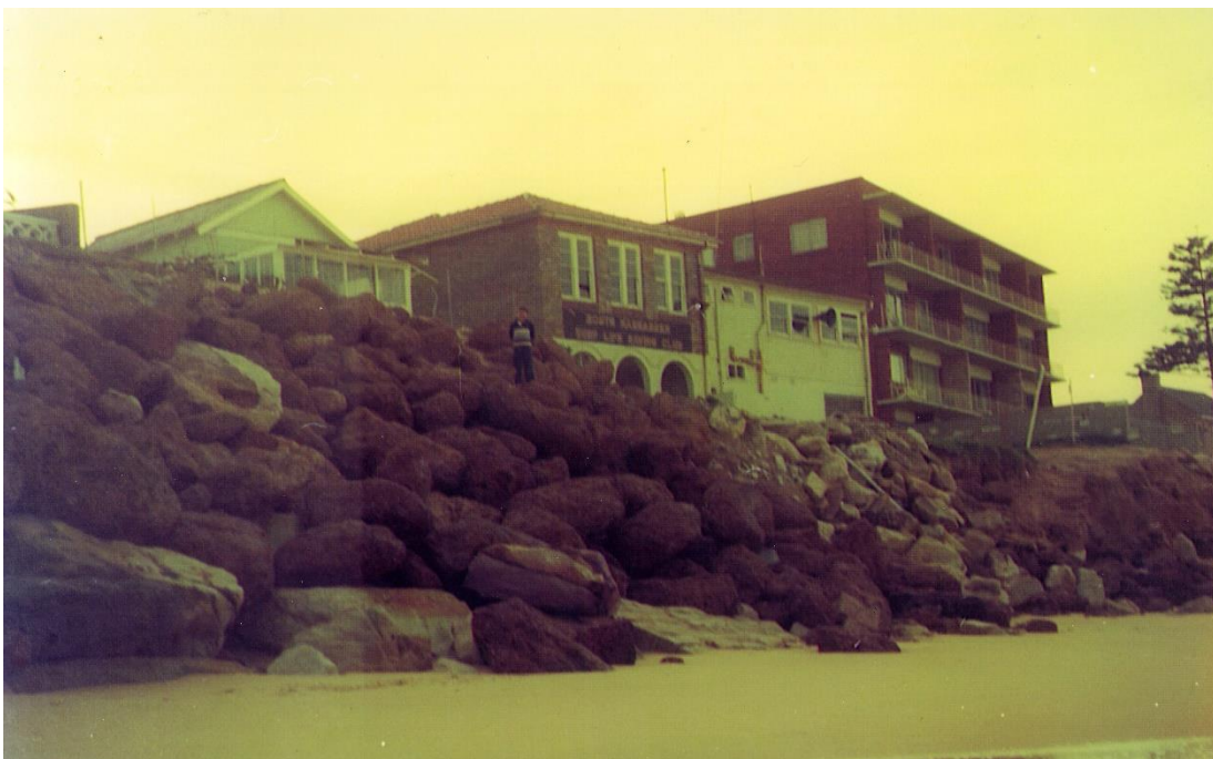
Figure 6: Protection works constructed at 1196 and former 1198 Pittwater Road in about 1975
