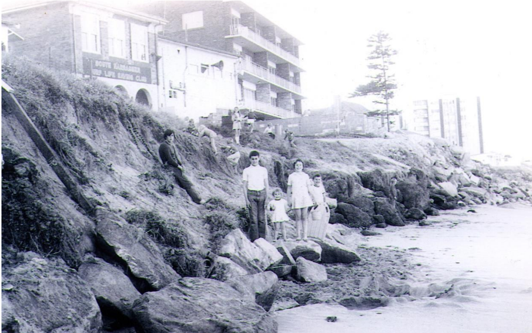
Figure 5: Exposure of protection works at 1194 and 1196 Pittwater Road in about 1974
