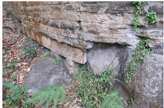
Figure 3.25 Sandstone outcrops with sandstone blocks laid over.
