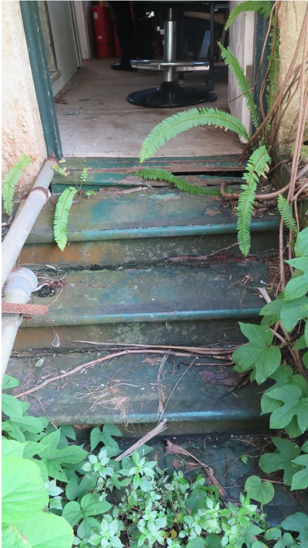
Figure 3.36 Caretaker's Cottage—granite steps form part of the front entry, with timber threshold in poor condition due to moisture.
