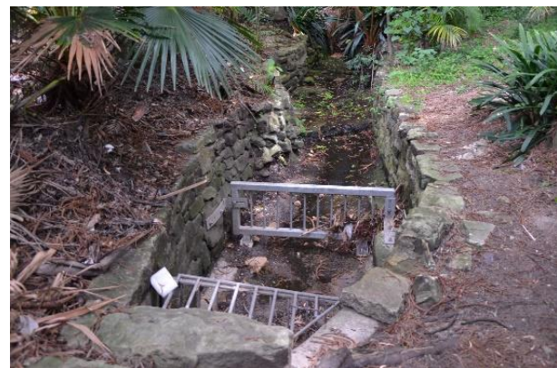
Figure 3.29 Metal gates (trash track) in the stone-lined creek to prevent the flow of debris into stormwater.
