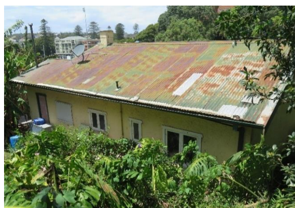
Figure 3.9 View of the Caretaker's Cottage showing the corrugated gabled roof.
