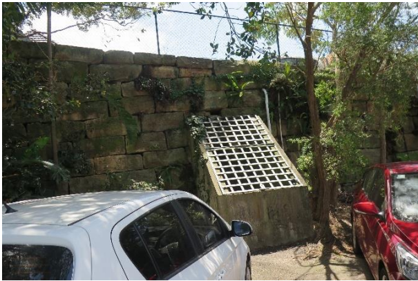
Figure 3.91 Raglan Street retaining wall with guard covering the stormwater line under the road.
