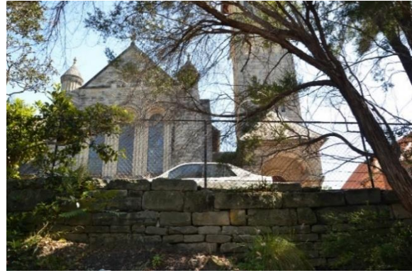
Figure 3.11 View of retaining wall to Raglan Street with various coursing of sandstone blockwork and chainwire fence above. (Source: Ari Anderson, December 2020)
