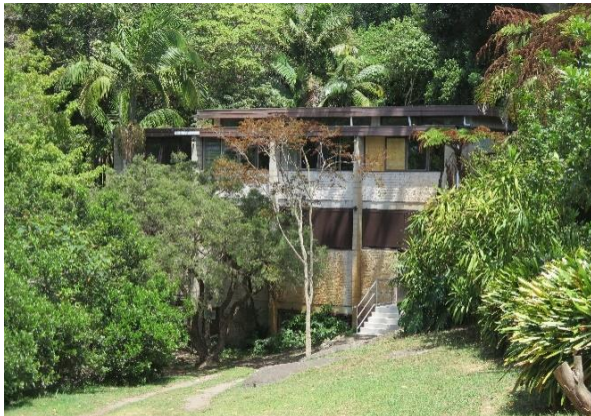
Figure 3.67 View of the east elevation of Fairlight Manly Scout Hall, a two-three storey concrete-framed building with face brickwork walls.
