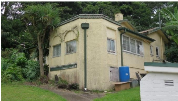
Figure 3.32 Southeastern corner of the Caretaker's Cottage showing the infill verandah extension.
