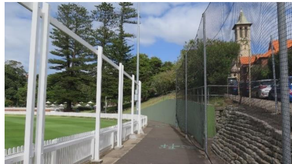
Figure 3.74 Sandstone retaining wall along the northern boundary, with the timber picket fence defining Manly Oval at left. Metal chainwire ball catching fence at right (Source: GML, December 2020)
