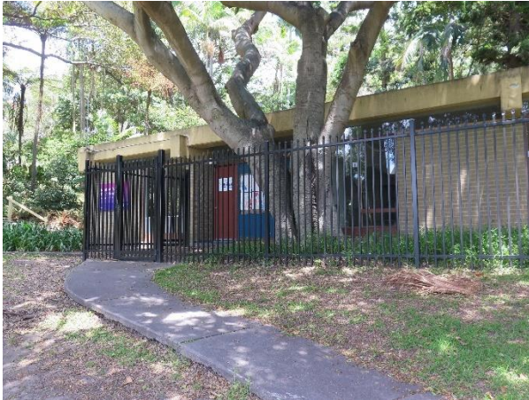
Figure 3.63 Kindergarten, east elevation, constructed in concrete frame with brick infill walls, within the valley among tree plantings. Dating to 1963.
