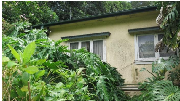
Figure 3.33 South elevation of the Caretaker's Cottage showing the timber-framed casement windows near the main entry. The cottage is surrounded by overgrown vegetation.
