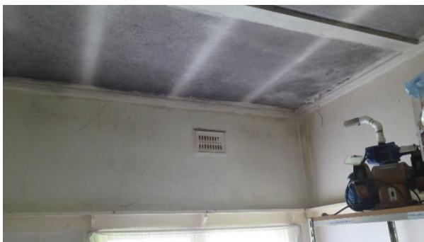
Figure 3.34 Evidence of mould in the fibrous plaster ceiling. Timber picture railings are fixed to walls in a number of the rooms.
