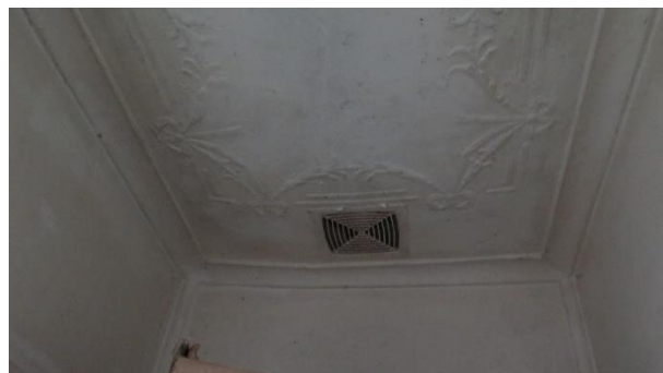
Figure 3.35 Interior of the Caretaker's Cottage showing the decorative fibrous plaster ceiling in the hall with air conditioning duct. The ceiling appears to be bowing due to water ingress.
