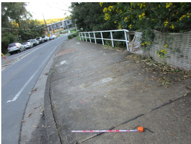
Plate 1: General view of the road bridge overlying the headwall, looking N.
