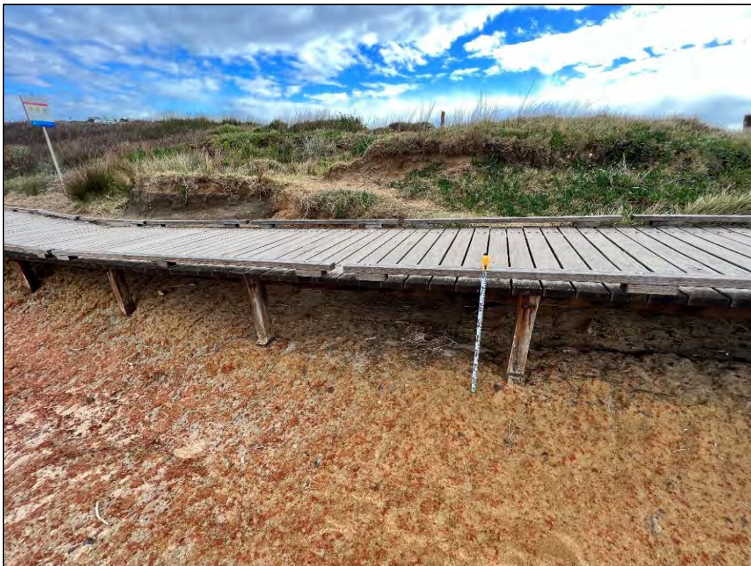
Plate 12: View north of western section of Long Reef boardwalk showing the exposed underlying geology on the south side of the boardwalk, and disturbed sand dunes profile on the north side.
