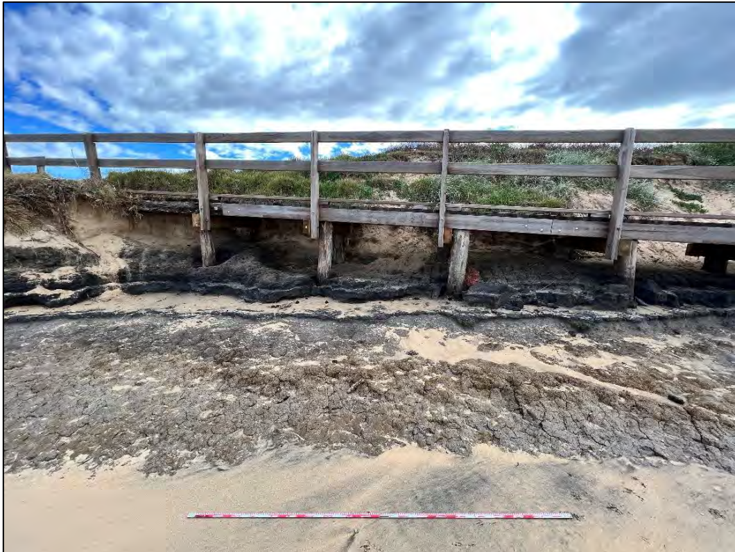
Plate 13: View north of eastern section of Long Reef boardwalk showing the exposed underlying geology on the south side of the boardwalk, and disturbed sand dunes profile on the north side.
