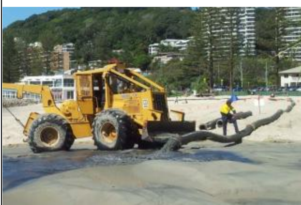
Sand being pumped along temporary pipe on beach, Burleigh, Qld Australia. (Image obtained from SMEC Jimmy's Beach Review of Management Options, March 2015)
