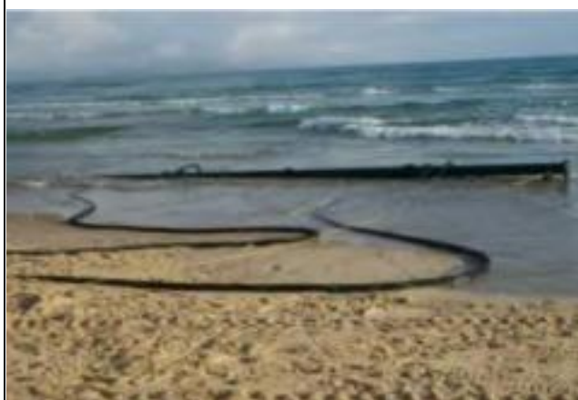
Noosa trial Sand Shifter in operation (unit buried). (Slurry Systems Marine)
