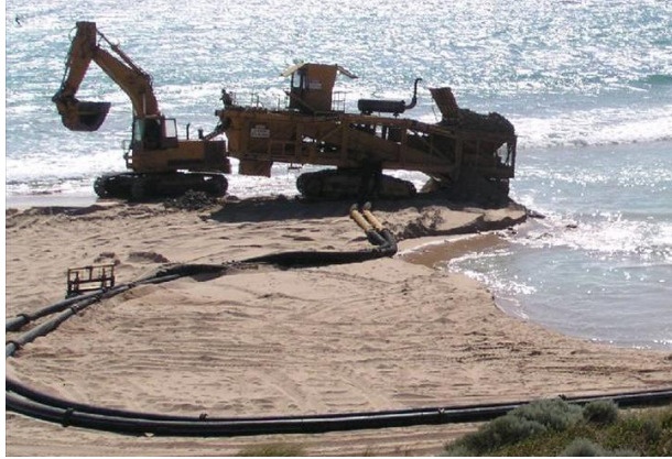
Sand is loaded in tracked mobile hopper and pumped, via temporary pipeline on beach surface, Dawesville WA
