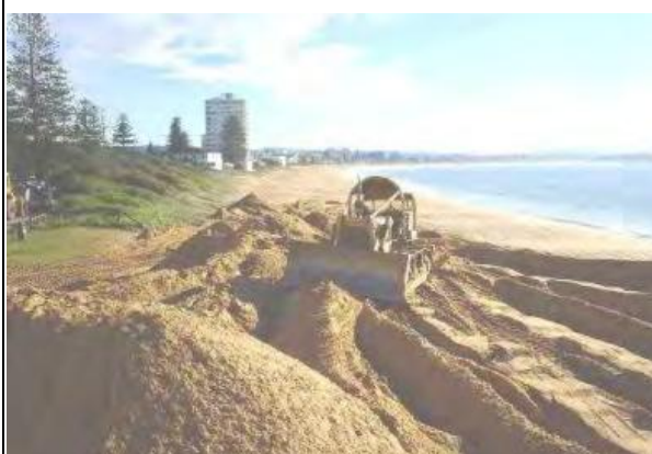
Placement and spreading of sand at Collaroy-Narrabeen Beach
