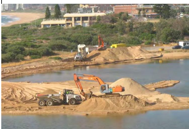
Sand extraction and transport via excavators and tip trucks
