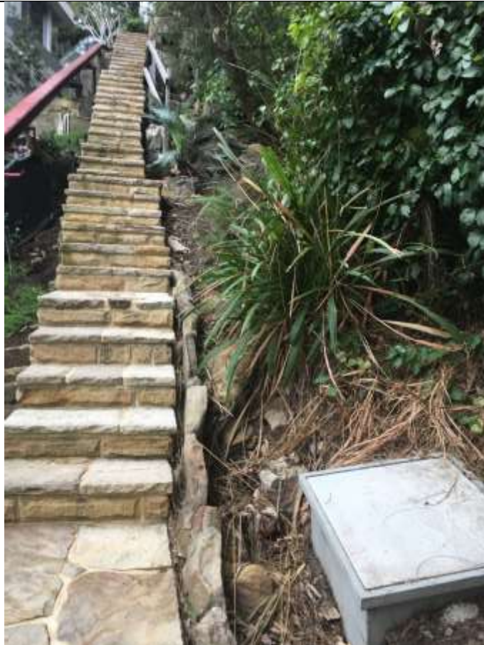
17. Showing stormwater pit looking up. Fall hazard on right (2.5m)
