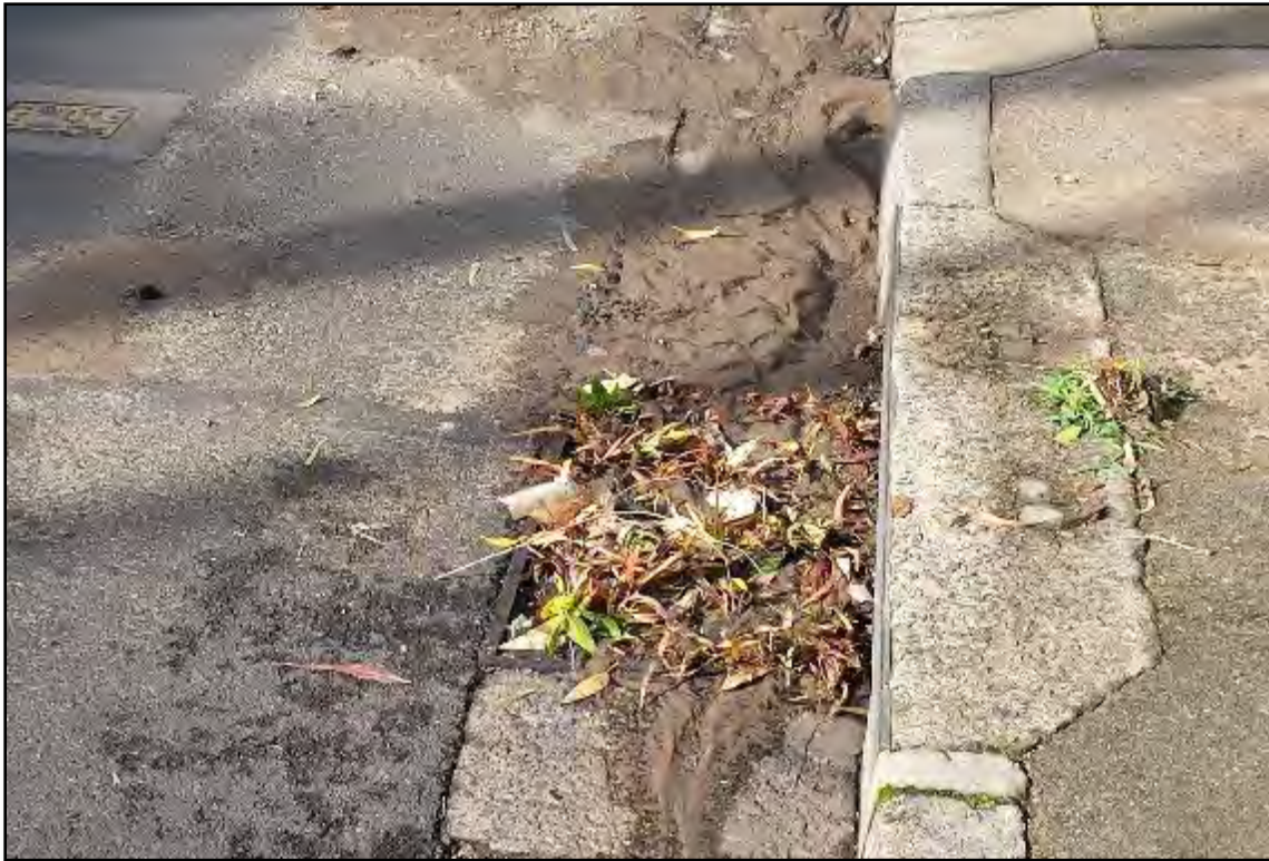
Plate 12 Typical blockage of a stormwater pit
