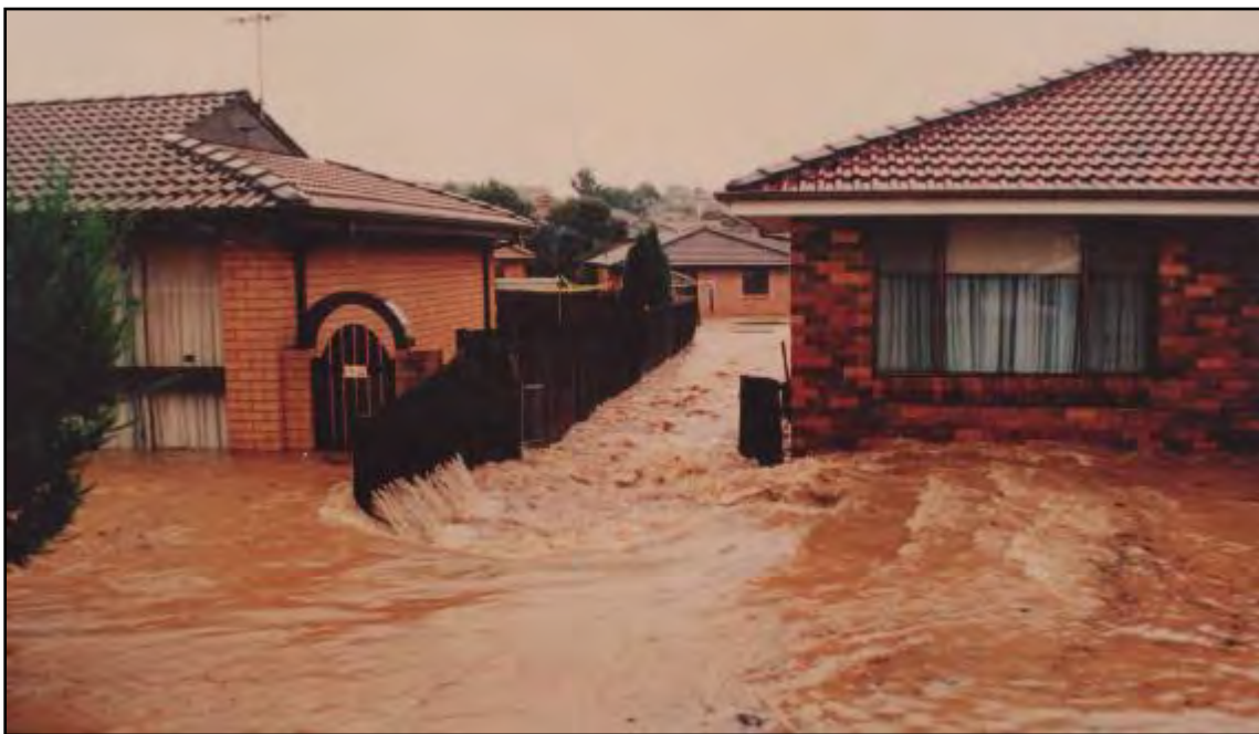
Plate 13 Example of fence causing a notable impediment and redistributable of overland flows
