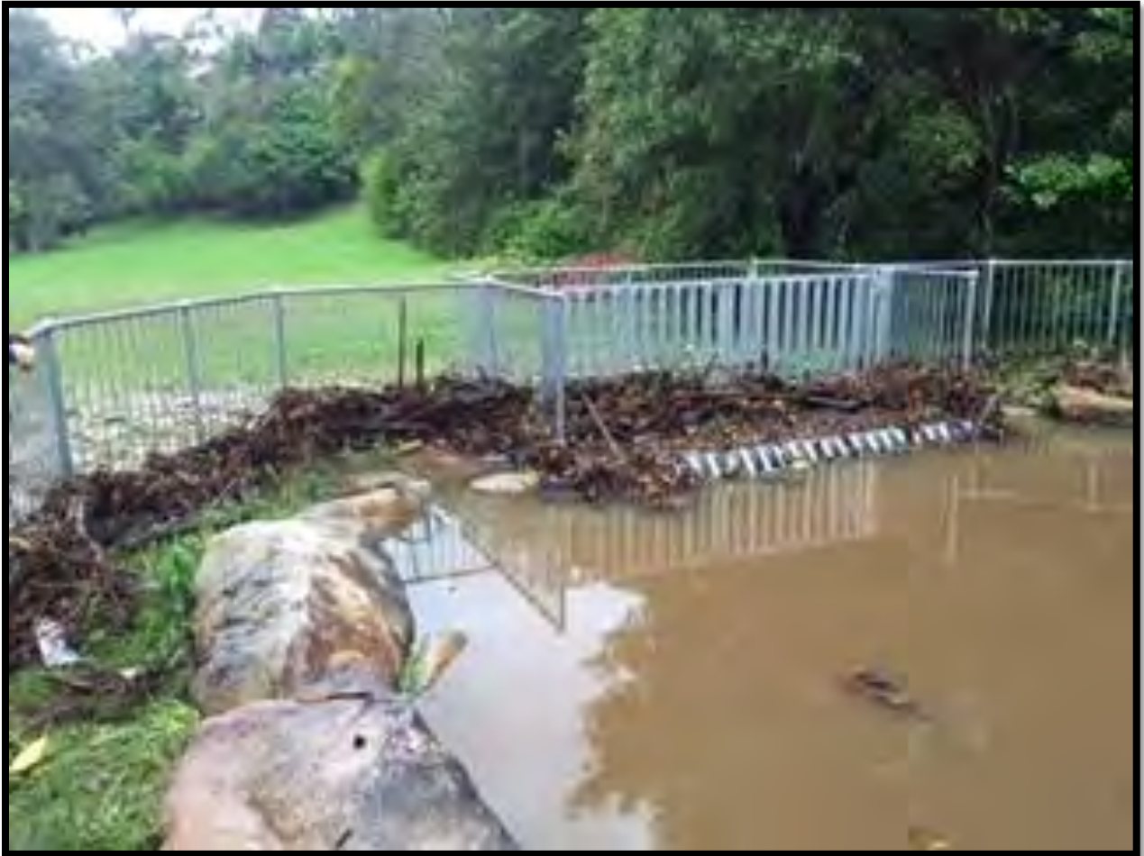
Plate 10 View showing build-up of debris on the upstream side of the trash rack at the Howell Close culvert during the 2012 flood
