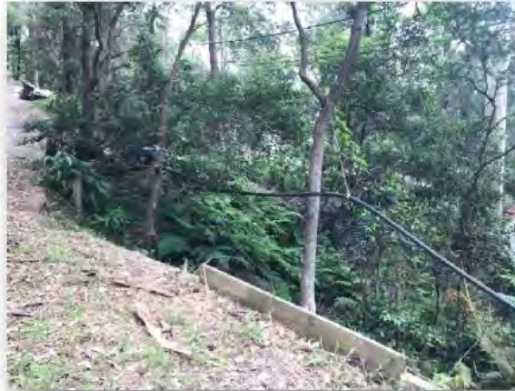
Photo 2-3: Small Bore Water Supply fixed to trees
