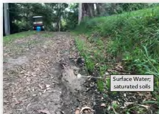
Photo 2-6: Evidence of surcharge from poorly performing on-site disposal
