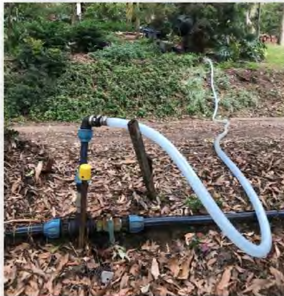
Photo 2-4: Tank Filling from Small Bore Pipeline
