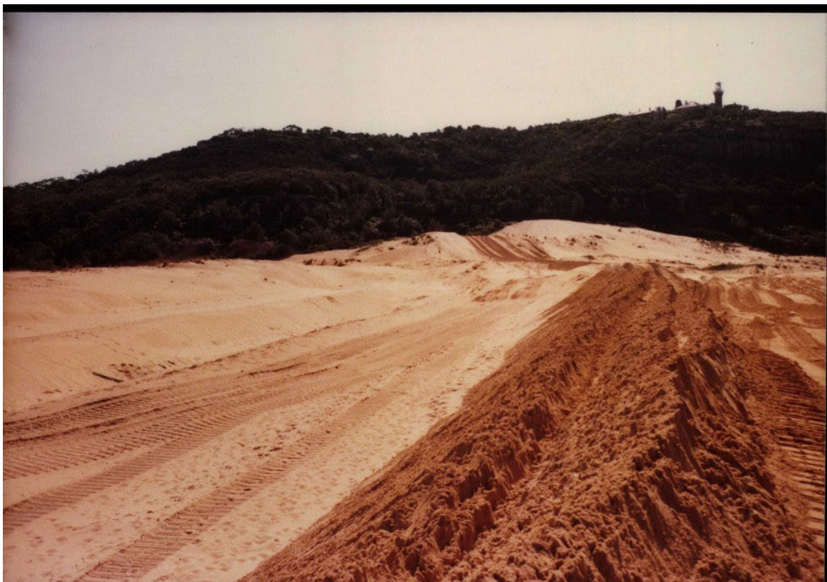
Plate 13: North Palm Beach showing modification to the sand dunes undertaken in 1984 to stabilise the dunes, c. 1984, image courtesy of Northern Beaches Council Local Studies Collection
