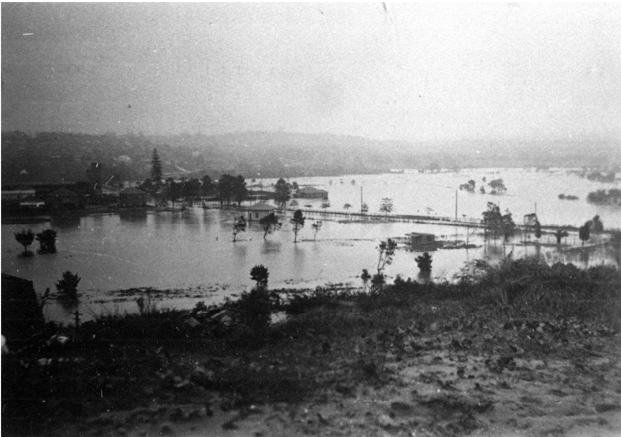
Figure 7: Historic flooding (1942) of Manly Lagoon at Pittwater Road, Queenscliff (Northern Beaches Council)
