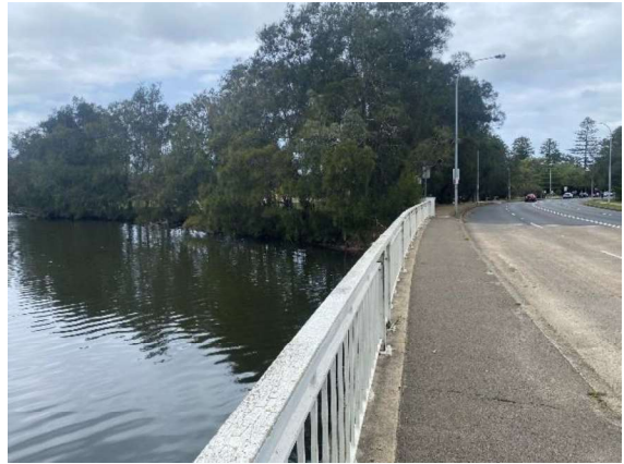
Figure 42: View south along existing pedestrian footbridge crossing Manly Creek
