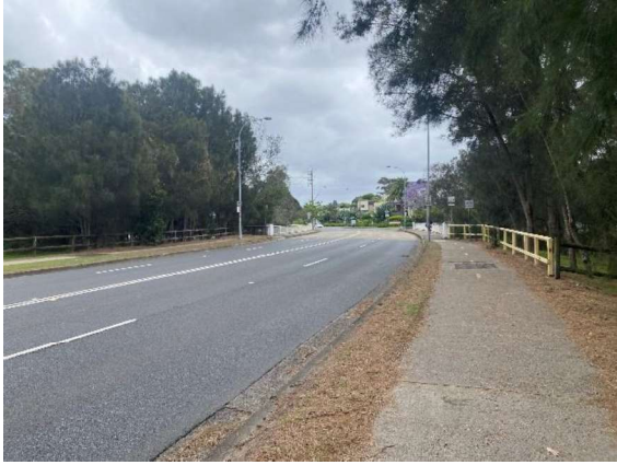
Figure 39: View north along Pittwater Road showing existing pedestrian footbridge, footpath, regrowth vegetation and the installation of below-ground services
