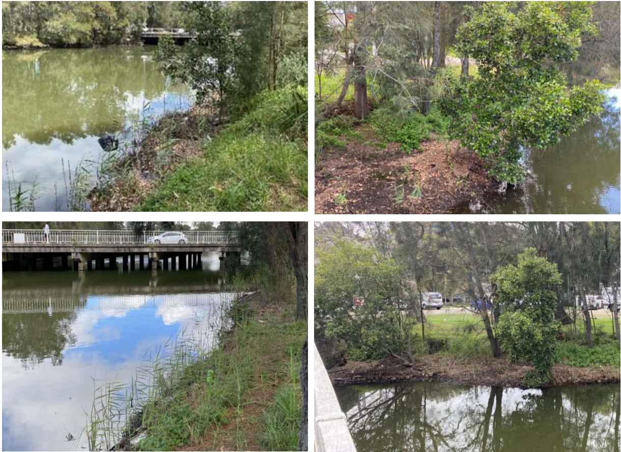
Figure 35: Grey Mangroves and Common Reeds occupying the intertidal zone north-east of the existing bridge
