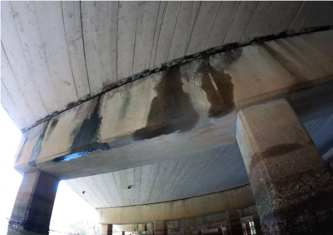
Figure 24: Potential microbat roosting habitat under bridge
