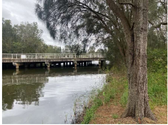
Figure 40: View south-west showing regrowth trees lining Manly Creek, existing pedestrian footbridge and approximate works area
