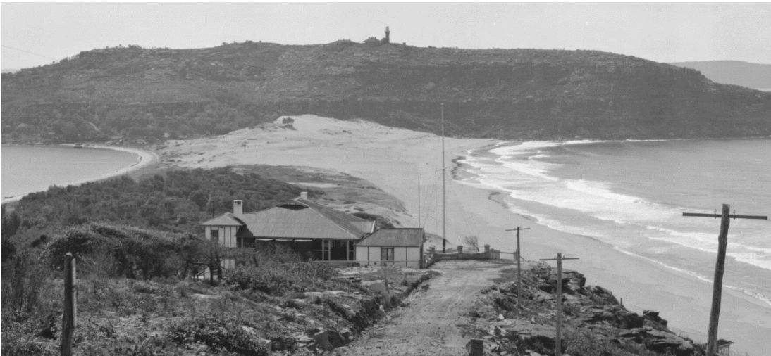
Figure 56: Detail from Panorama of Palm Beach showing the northern side (middleground) and Barrenjoey Lighthouse and Headland (background), EB Studios, 1917-46 (Source: National Library of Australia, PIC P865/207/11 LOC Nitrate store)
