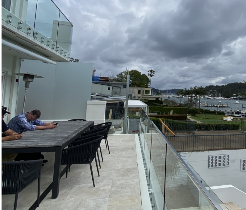
Figure 9: Existing ground floor balcony and privacy screening facing 18 Rednal Street
