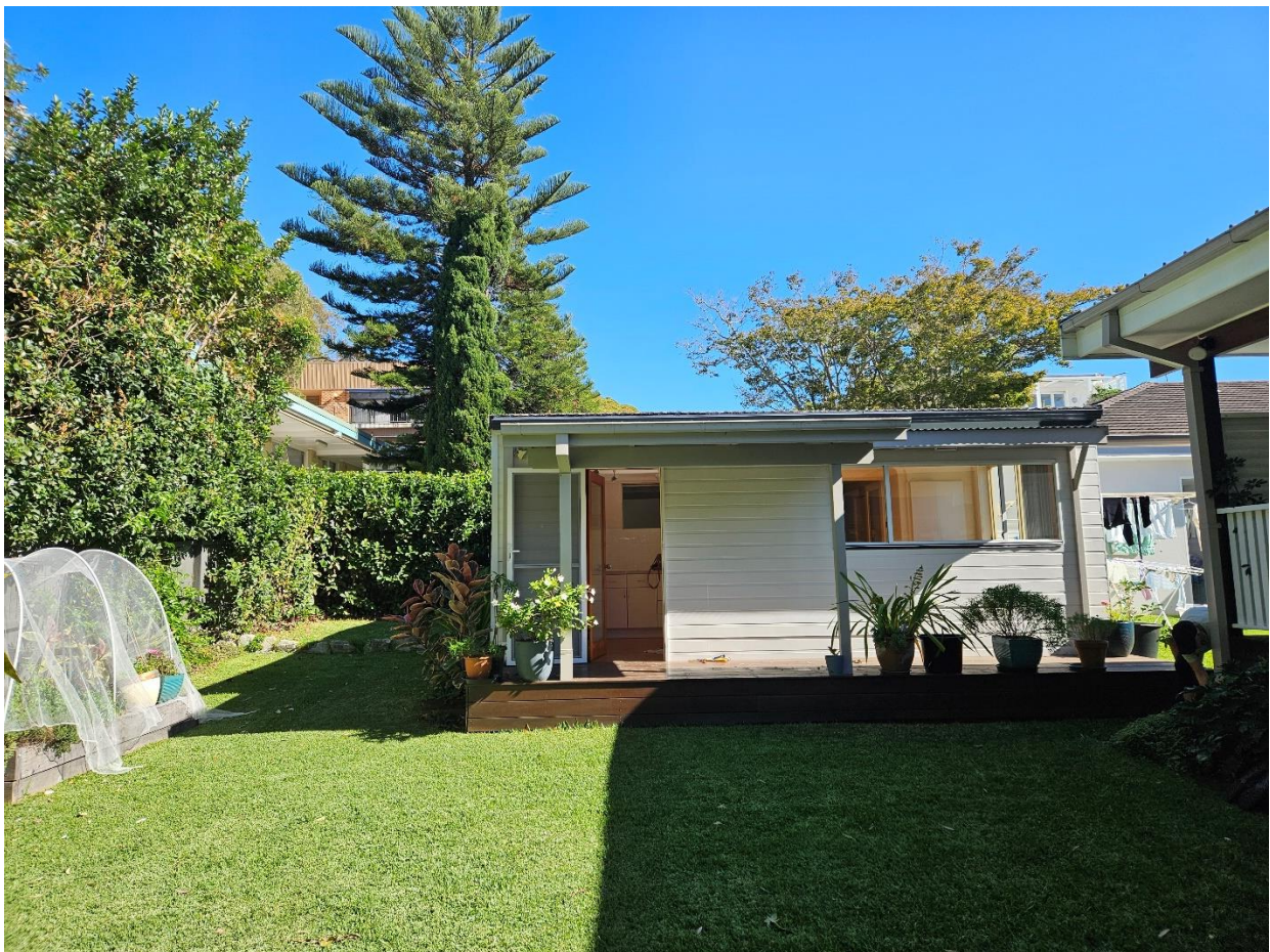
EAST VIEW LOOKING TOWARDS THE EXISTING STUDIO ENTRANCE AND THE LAUNDRY
