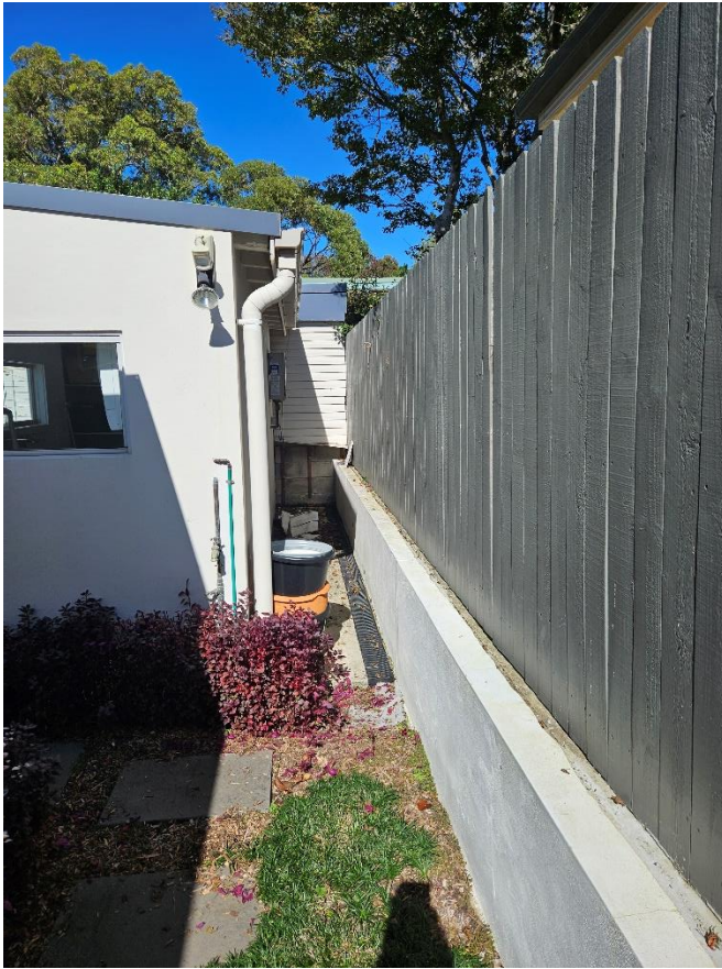
NORTH-WEST SIDE OF THE EXISTING LAUNDRY REAR AND NEW ENTRANCE TO THE GRANNY FLAT
