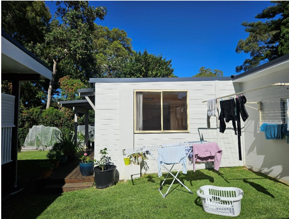
NORTH VIEW LOOKING AT THE SIDE OF THE STUDIO AND THE PROPOSED EXTENSION LOCATION
