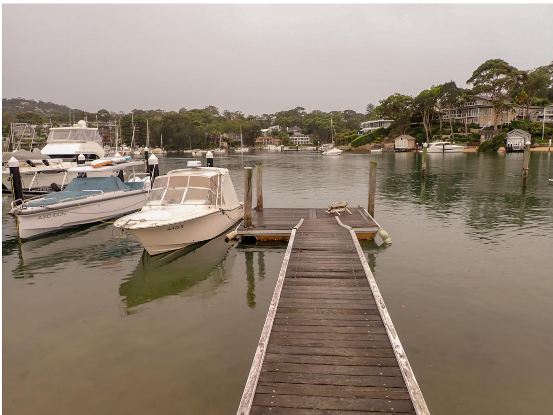
Photo 2. The existing timber jetty, ramp, pontoon, pontoon stabilising piles and fender pile – all of these structures are proposed to be removed.
