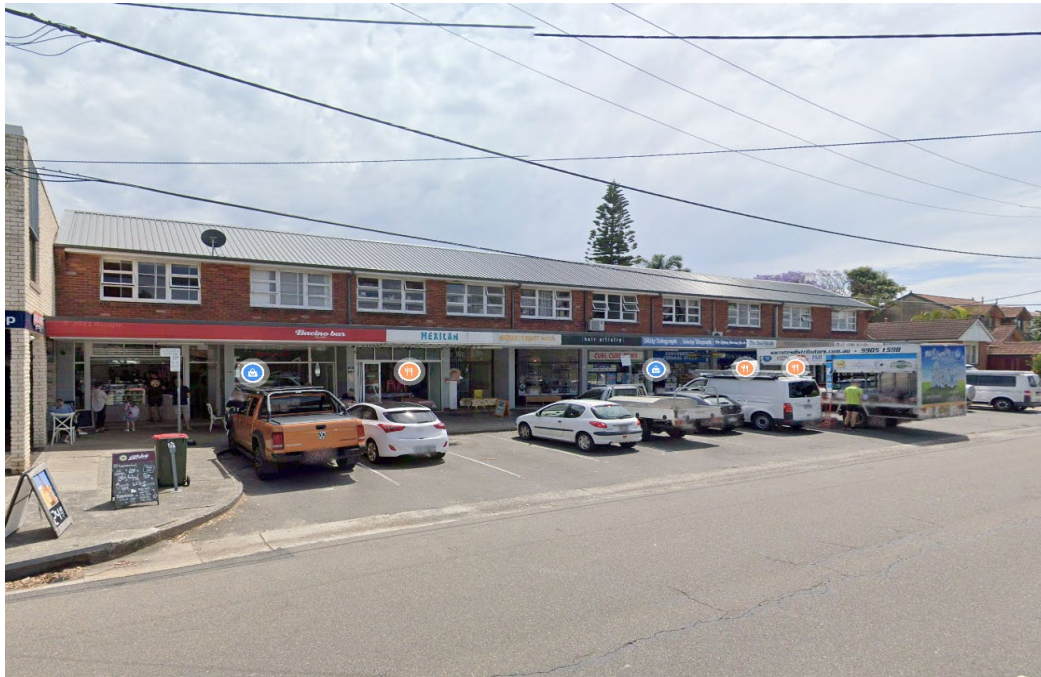
The subject site as viewed from Pitt Road
