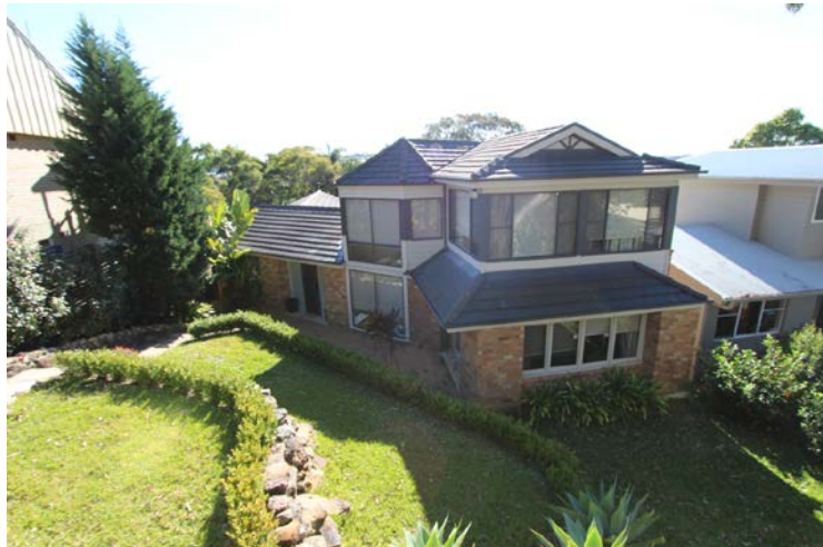
Fig 3: View of the dwelling from the Southern (front/street) side. ( Action Plans 2018 ).
