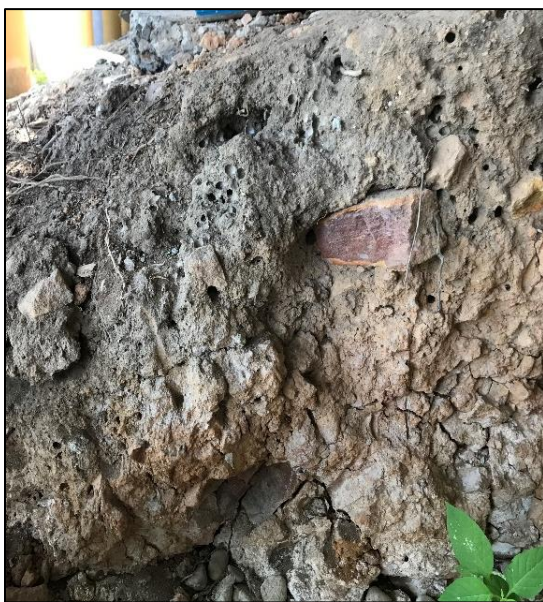
Photograph 3: View of the soil exposed under north end of the site house
