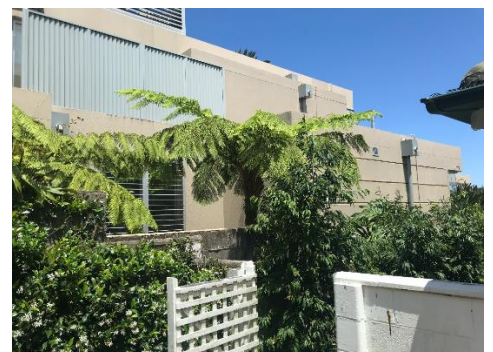
Figure 32: Existing privacy screen along western facade of 90 Lauderdale Ave (Source: Archer Office)
