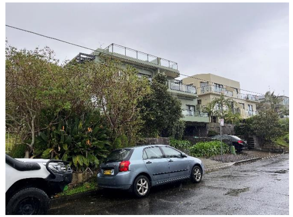
Figure 13: 14-14A Willyama Avenue, northeast of the subject site (Source: GYDE Consulting)
