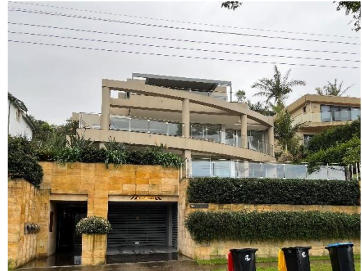
Figure 5: 90 Lauderdale Avenue, adjoining to the east (GYDE Consulting)
