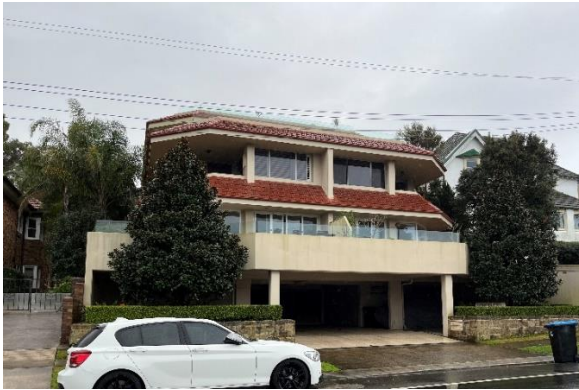
Figure 4: 94 Lauderdale Avenue, adjoining to the west (GYDE Consulting)
