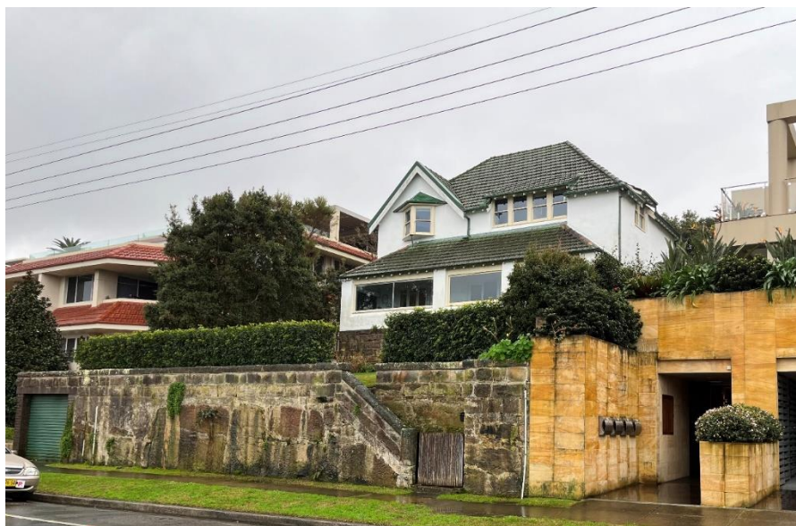
Figure 2: Existing dwelling house at Lauderdale Avenue (Source: GYDE Consulting)
