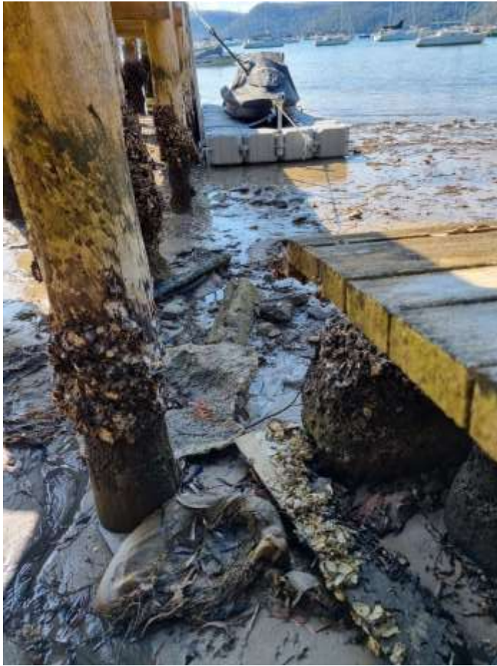
Figure 4 – Photo 3 of jetski pontoon at low tide, 24 December 2022
