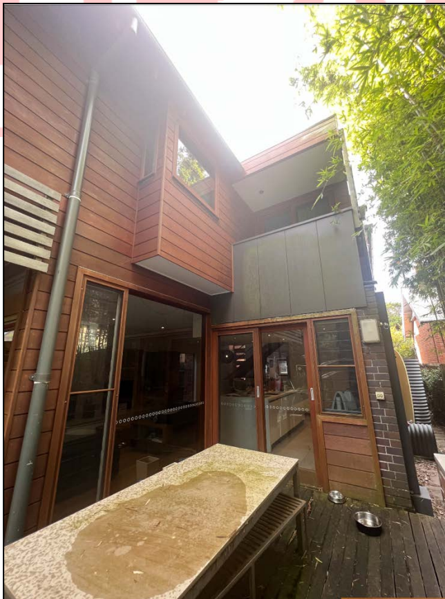
Figure 7: Deck area to be transformed into a dining room..
