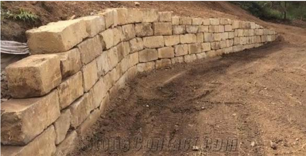
Sandstone retaining wall →
