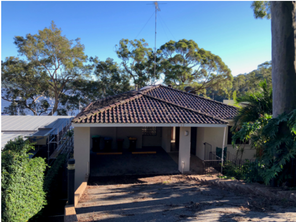
Photograph 1: The site and the existing steep driveway, partly within the road reserve and front carport and the house behind, viewed from the street.
