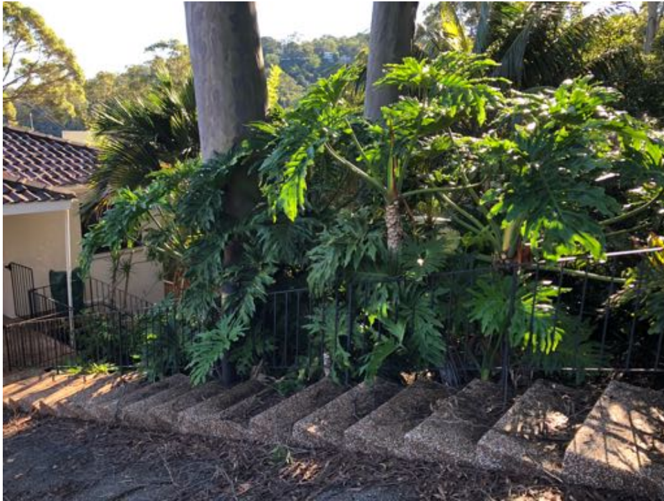
Photograph 5: The existing steps on the side of the driveway for access down to the house. The two existing spotted gum trees adjoin the front boundary of the site.
