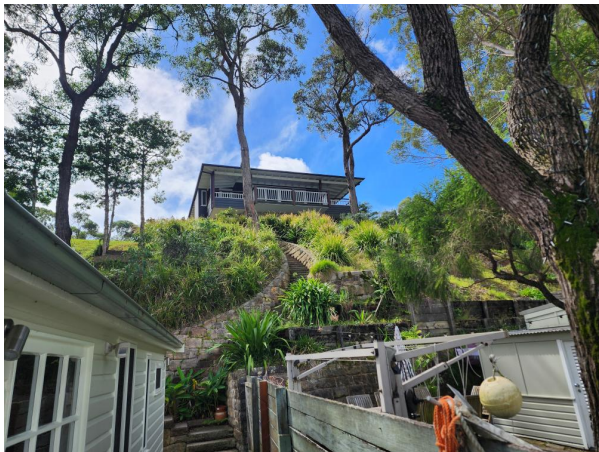
31 Sturdee Lane, looking North from foreshore
