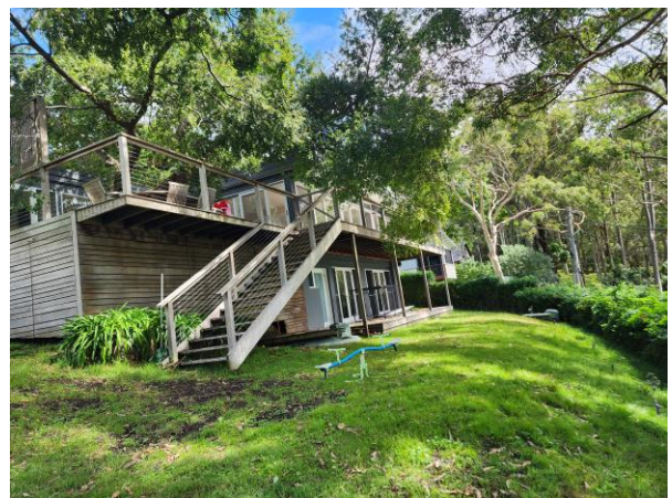
33 Sturdee Lane, looking South West
