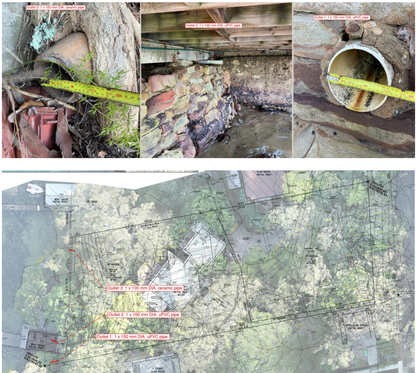
Figure 1 – Existing Stormwater Outlet Pipes
