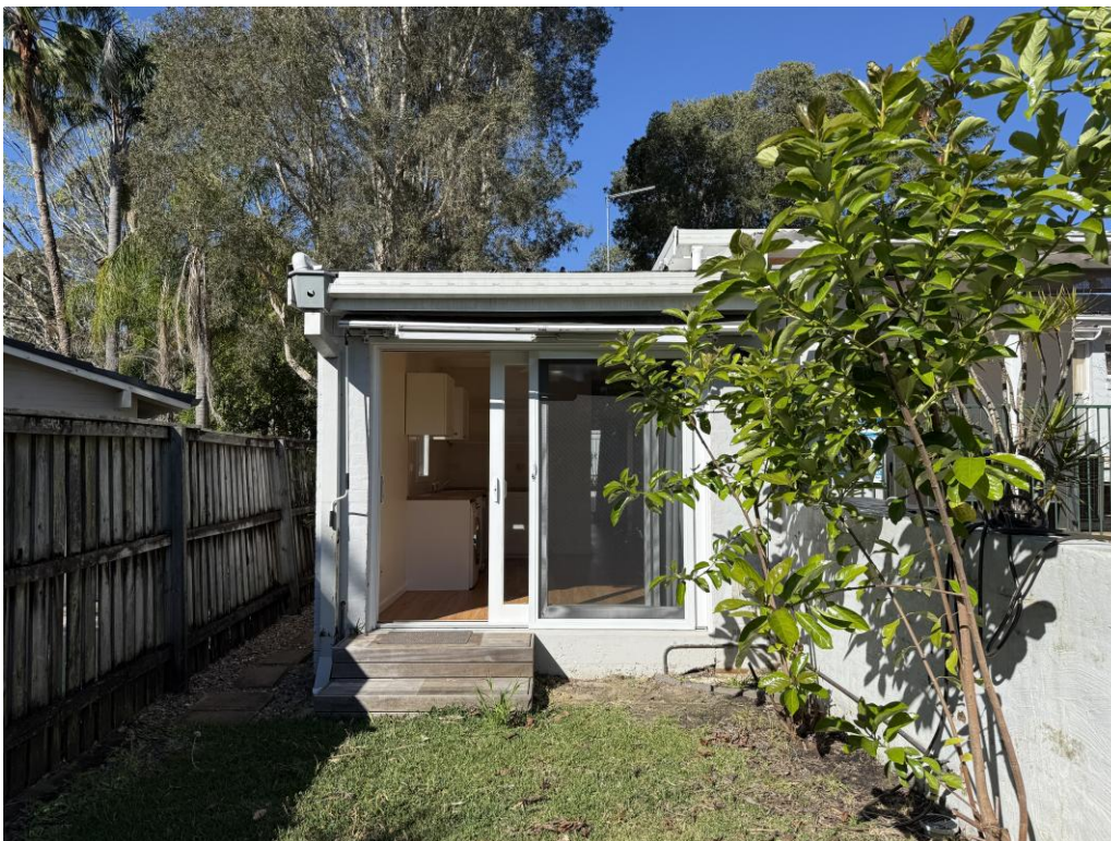
Figure 5: The existing workshop space, looking east.
