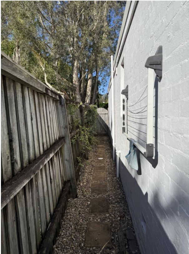
Figure 6: The northern elevation of the garage/habitable space conversion, looking east.
