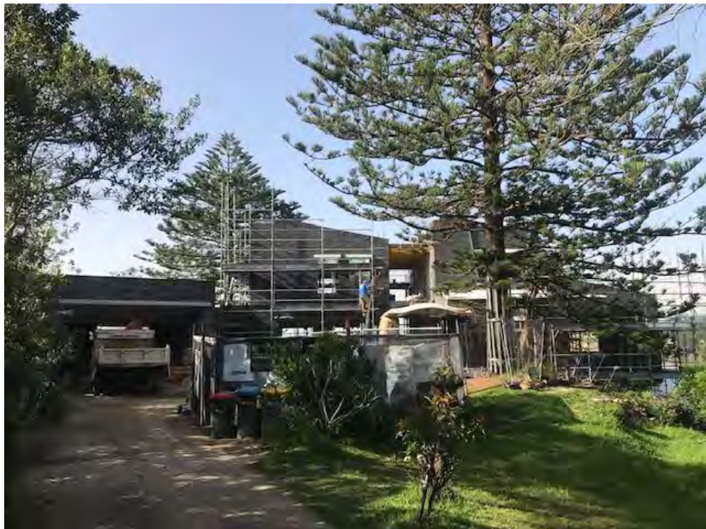
The dwelling under construction viewed from adjacent to the S/W facing wall of No.43 Marine Pde.
