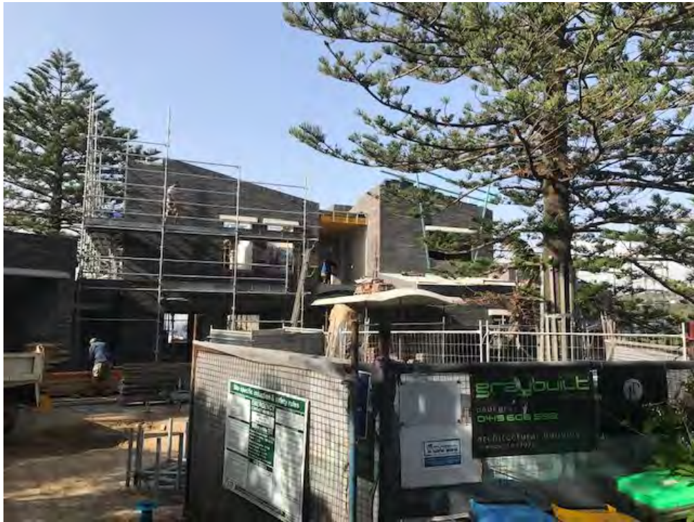
The dwelling under construction viewed from the top of the driveway.
