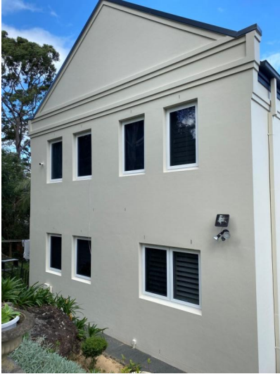
FRONT FACADE - NORTHERN ELEVATION
