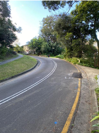
VIEW ALONG JENNER STREET LOOKING EAST
