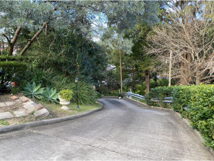
VIEW OF EXISTING REAR DRIVEWAY FROM REAR GARDEN
