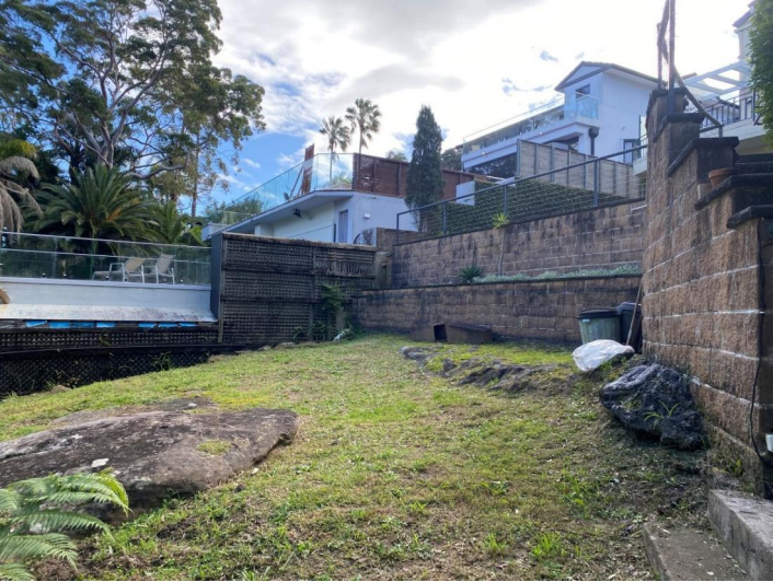
VIEW OF REAR RETAINING WALLS AND SOFT LANDSCAPING IN REAR GARDEN
