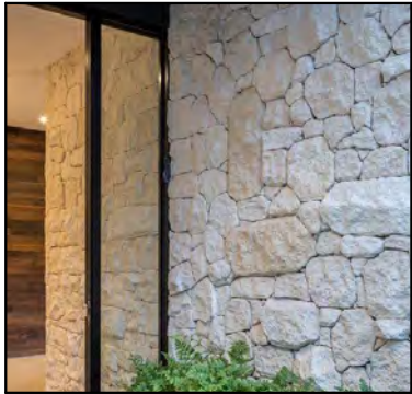
5 - STONE FEATURE CLADDING: FINISH TBC BY CLIENT
