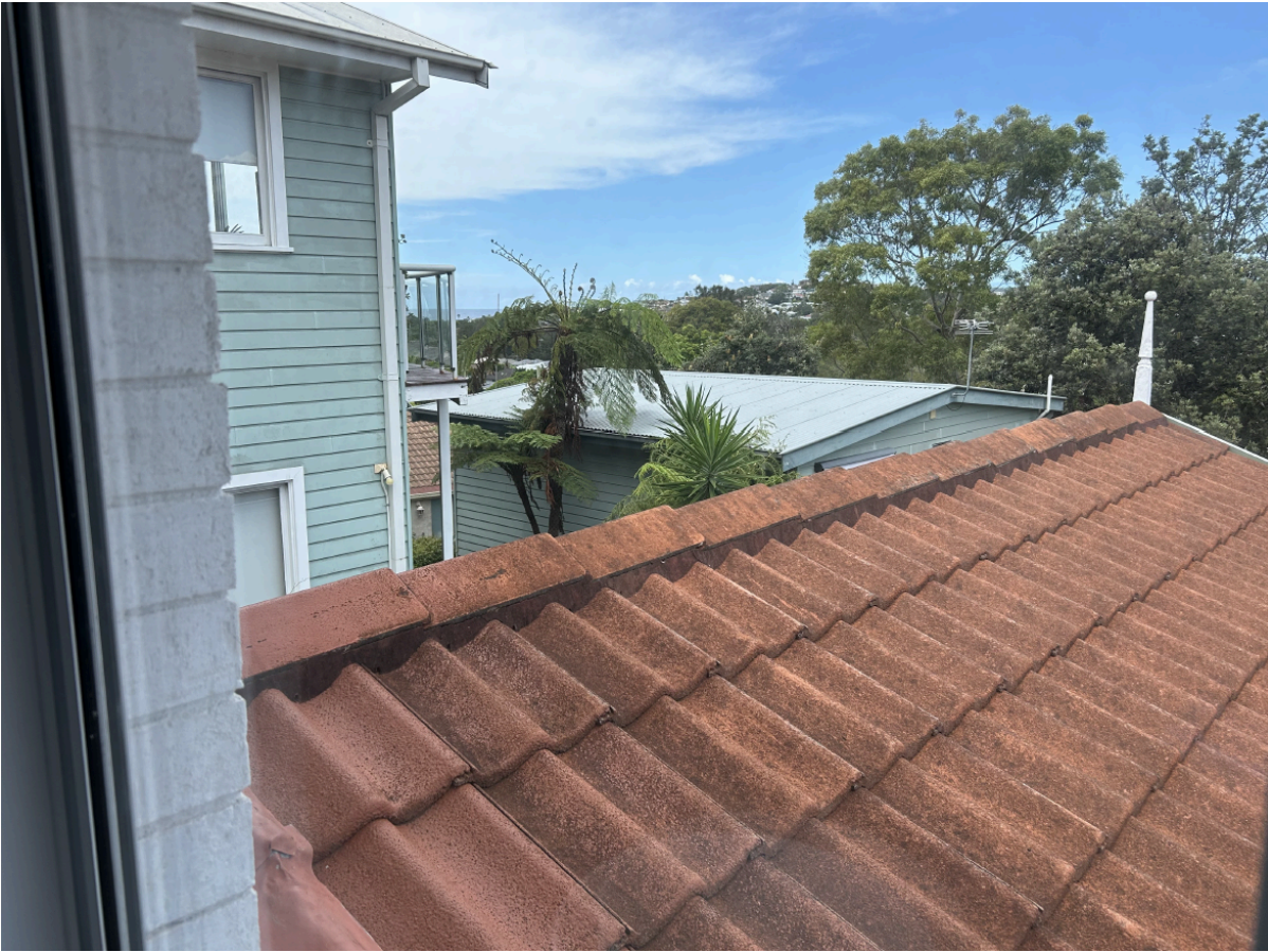
Figure 5 - View from First Floor Bedroom of 16 Rabaul Road looking south-east (toward the subject site). Taken on 11 Febuary 2025.
