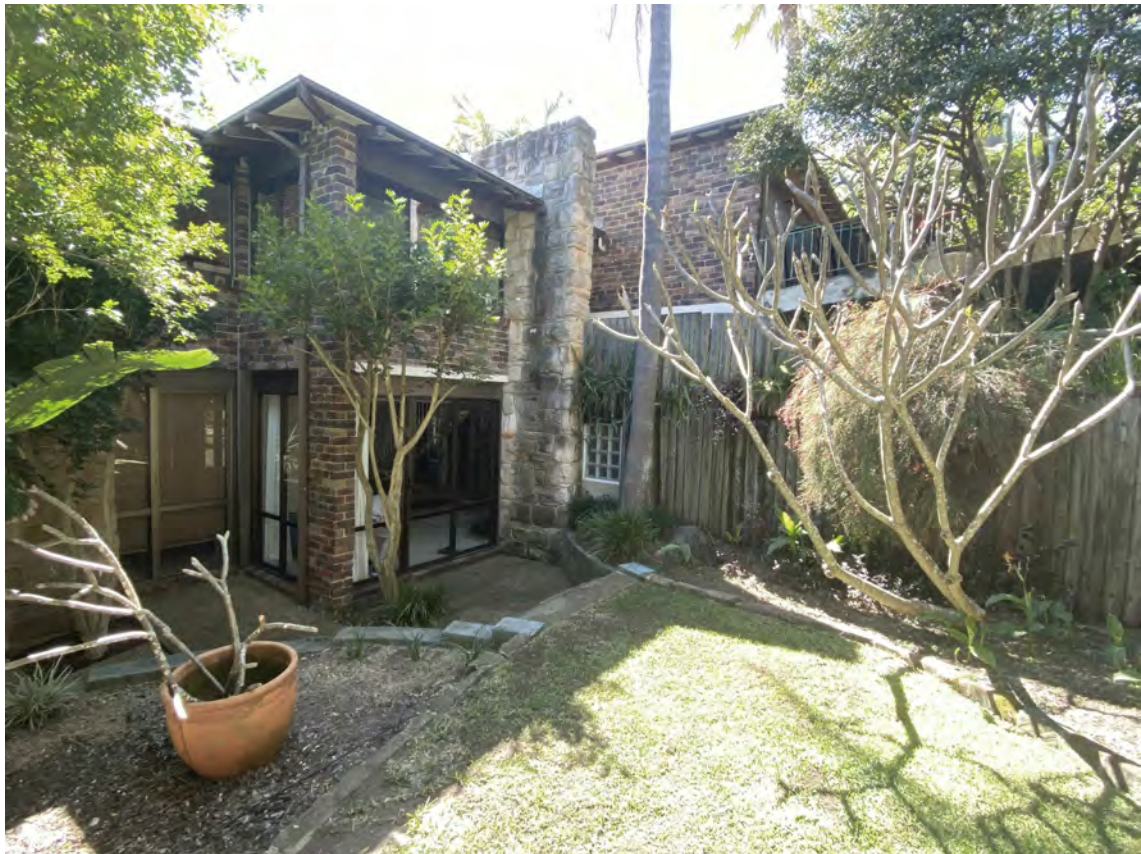
EXISTING VIEW - VIEW FROM GARDEN FACING NORTH EAST
