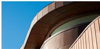
G - COPPER STYLE ROOFING
