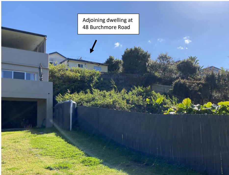
Figure 13. The location of the adjacent dwelling to the north and the existing dense vegetation immediately adjoining the subject dwelling
