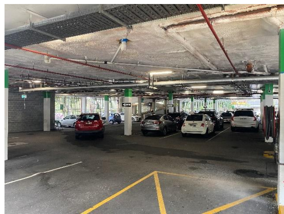
View of existing carparking area for the proposal
