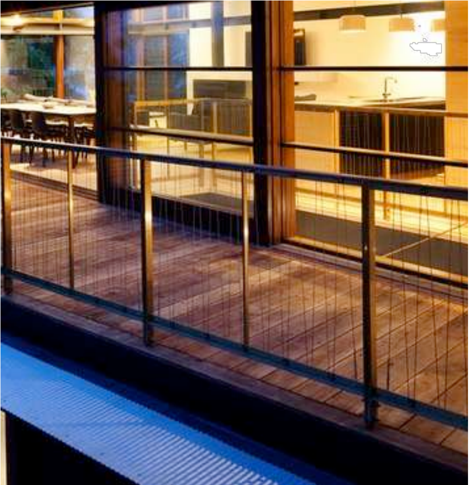
BALUSTRADE - STEEL WITH TIMBER RAIL
