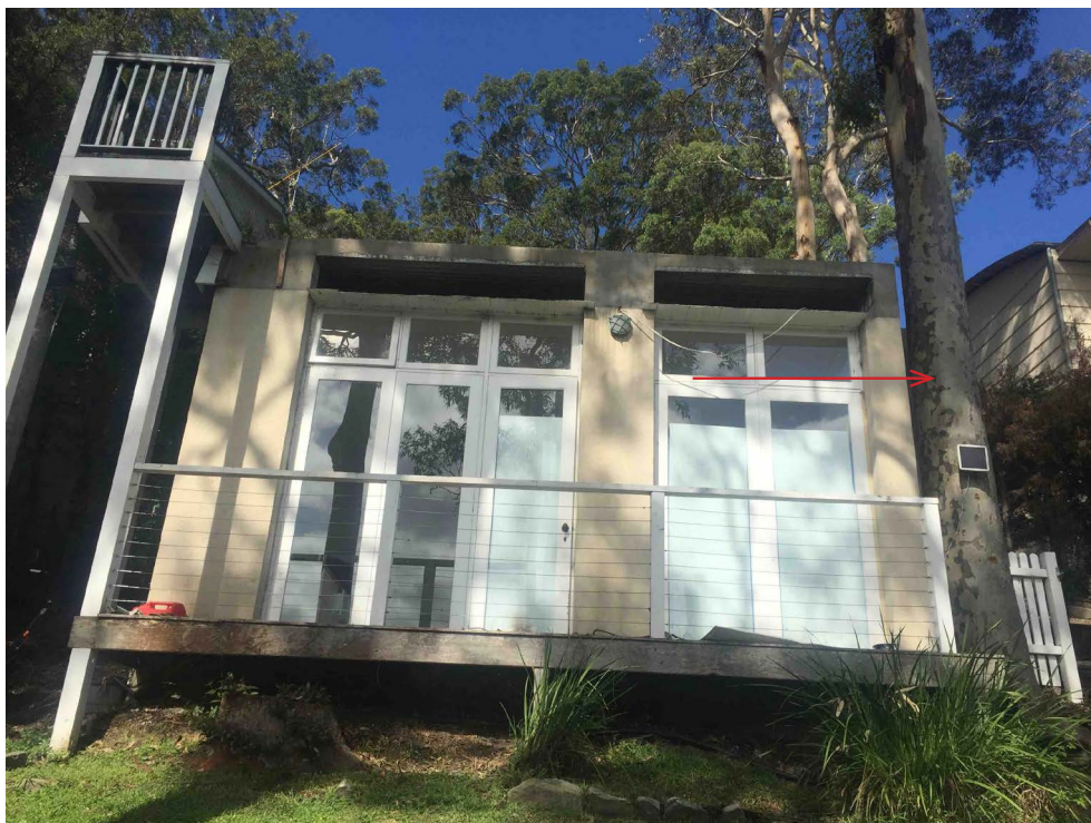
Figure 3: Photograph viewing east at the studio with the garage concrete slab above. The trunk of Tree No. 1 (Spotted Gum) is visible to the right hand side. (Photo: J Willis)
