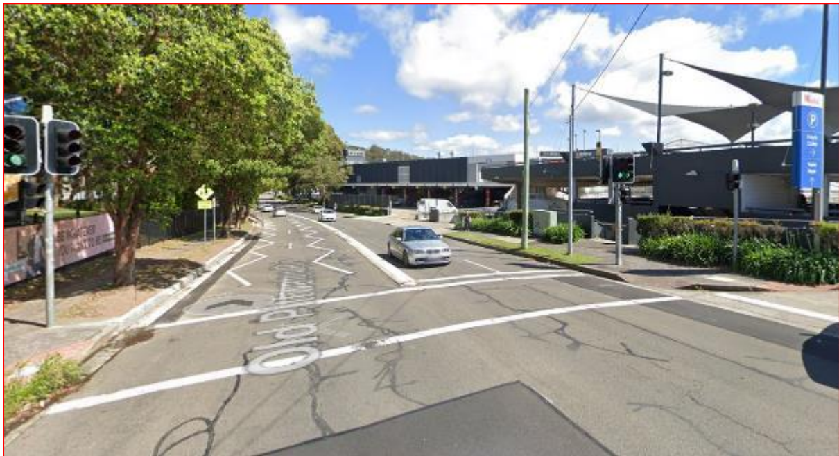
FIGURE 11: OLD PITTWATER ROAD – WESTFIELD SHOPPING CENTRE PEDESTRIAN CROSSING
