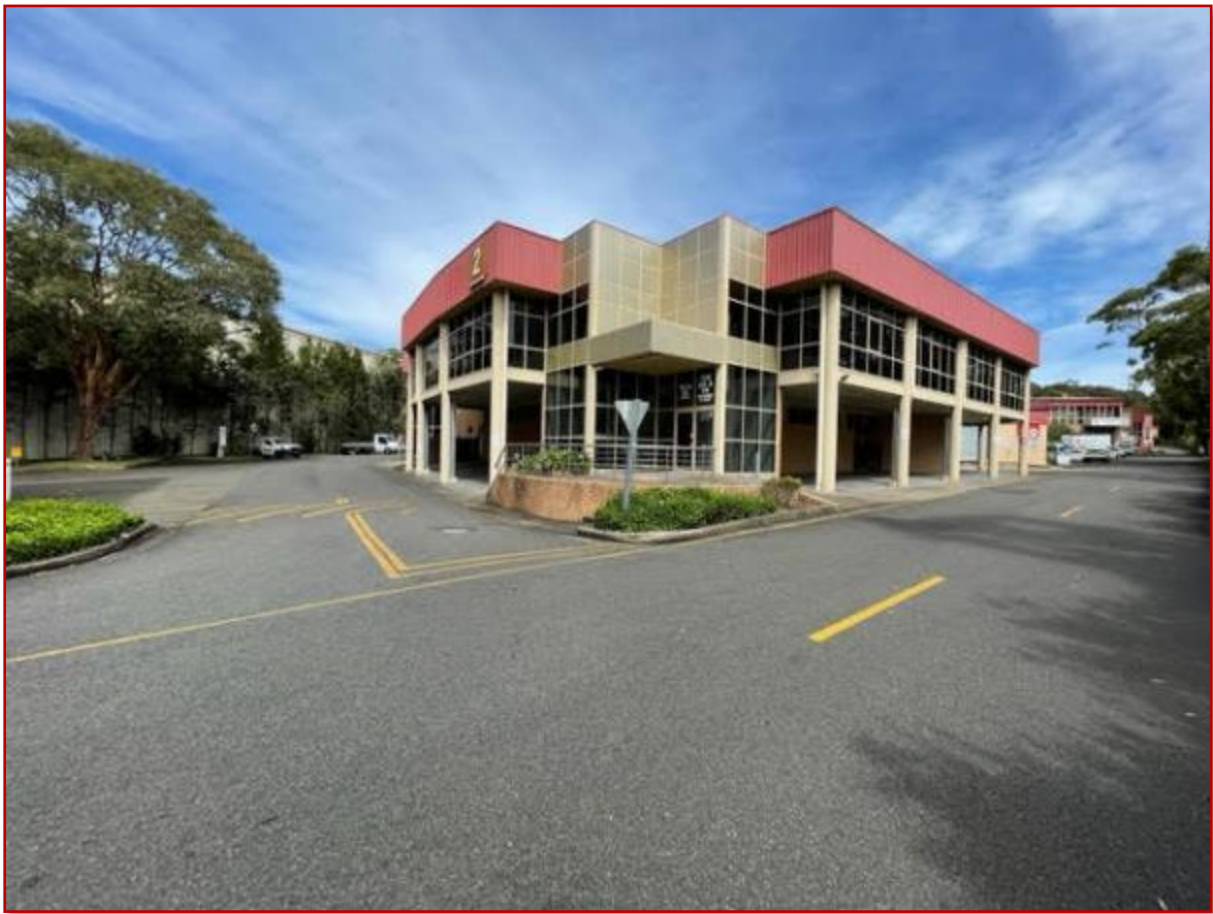
FIGURE 24: TYPICAL INTERSECTION WITHIN THE FACILITY WITH APPROPRIATE TRAFFIC MANAGEMENT FEATURES
