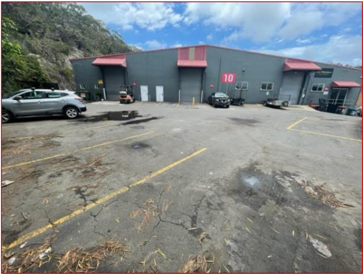
FIGURE 8: PARKING WITHIN 106 OLD PITTWATER ROAD COMPLEX
