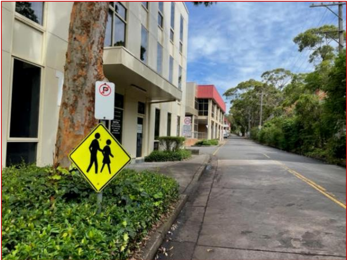
FIGURE 21: MAIN ACCESS ROAD WITHIN THE FACILITY
