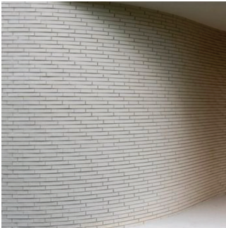
CURVED BRICKWORK WALLS
