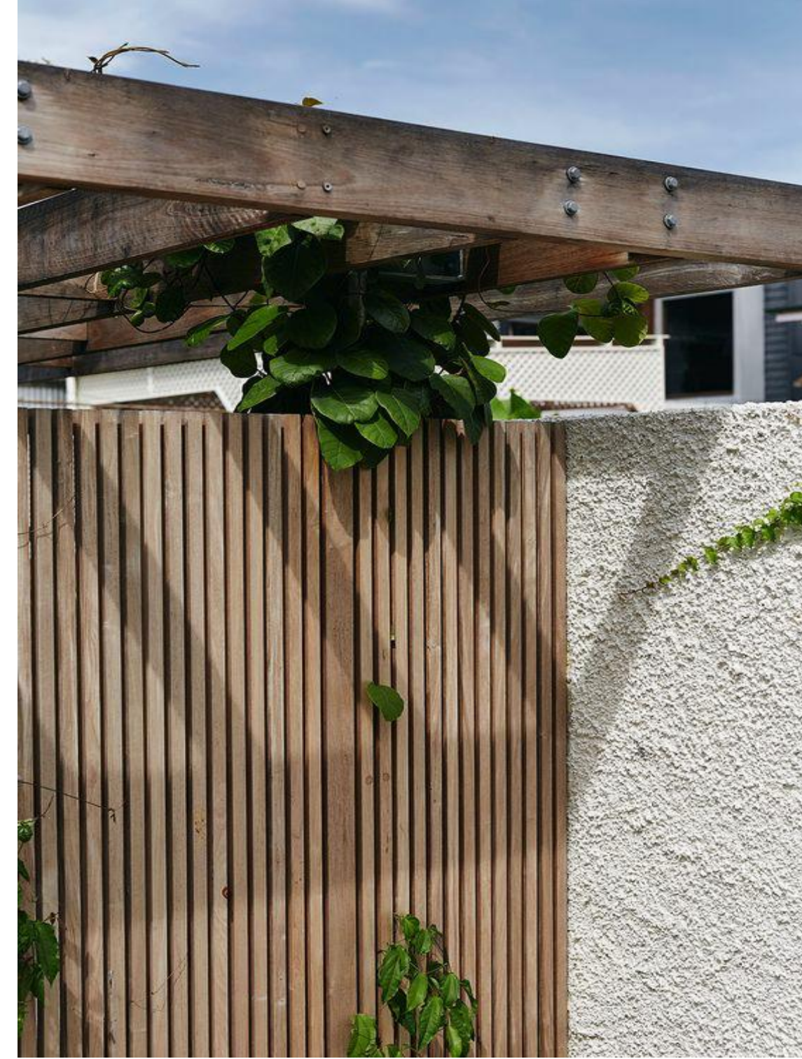
3 VERTICAL TIMBER BATTENS
