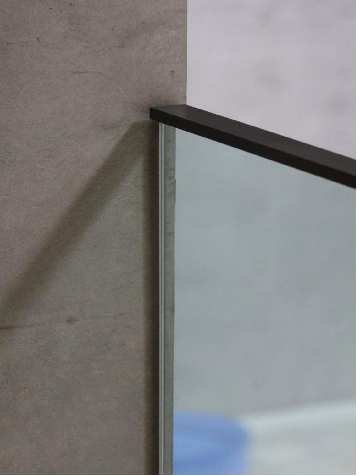
4 FRAMELESS GLASS BALUSTRADE WITH BRONZE CAPPING
