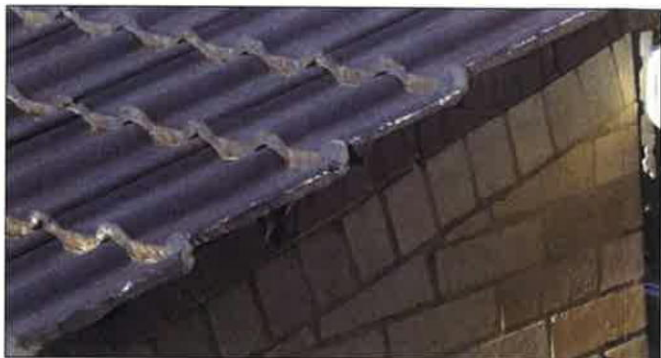
EXISTING ROOF TILES RETAINED
