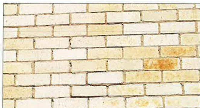
EXISTING BRICKWORK RETAINED
