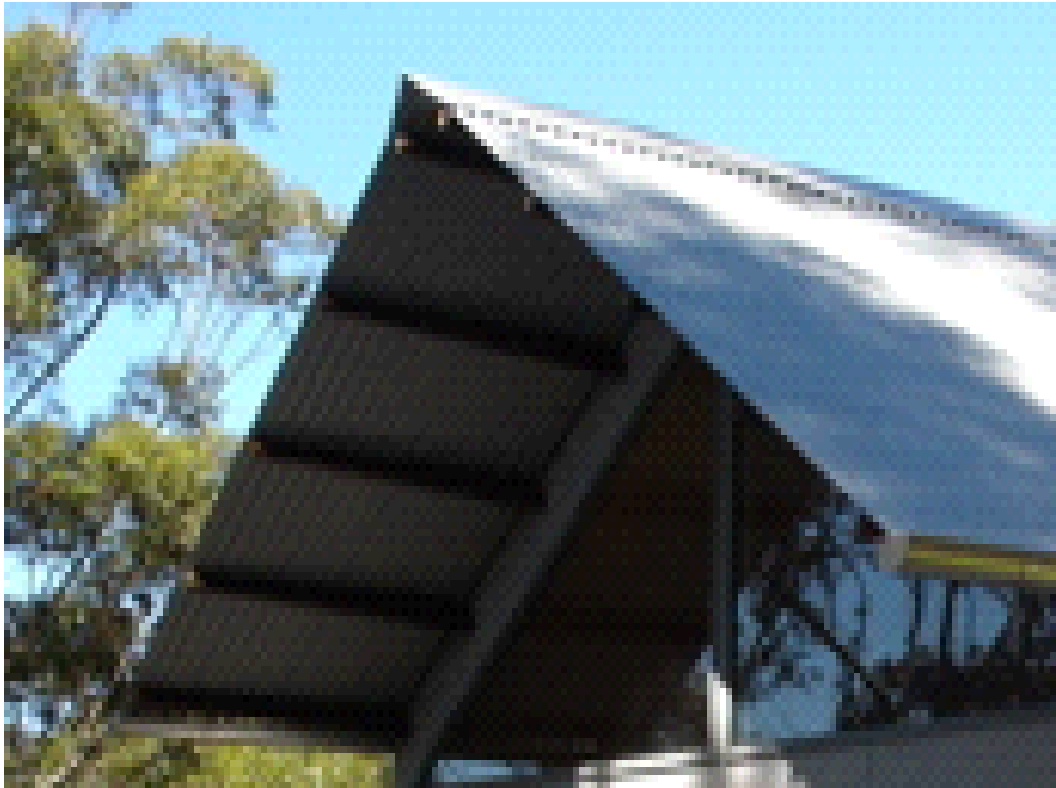
CORRUGATED COLOURBOND ROOF
