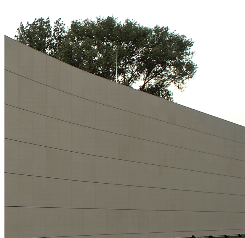
NEUTRAL COLOURED LANDSCAPE AND BASEMENT WALLS
