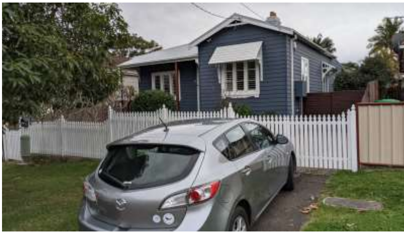
Looking at No.4 from Burchmore Road
