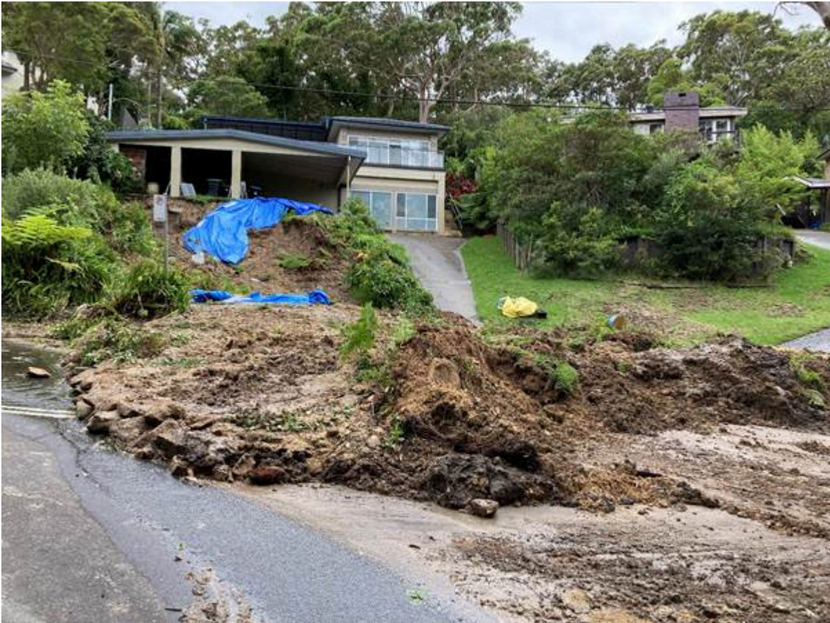
Landslide March 2022, Lower Plateau Road, Bilgola Plateau
