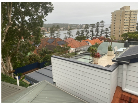
Rear 1 st floor of 16 Margaret St east with SE view across No.14
