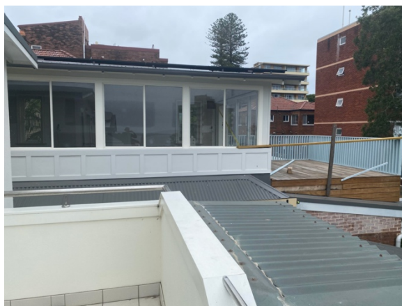
Rear 1 st floor of 16 Margaret St looking NE to No.18
