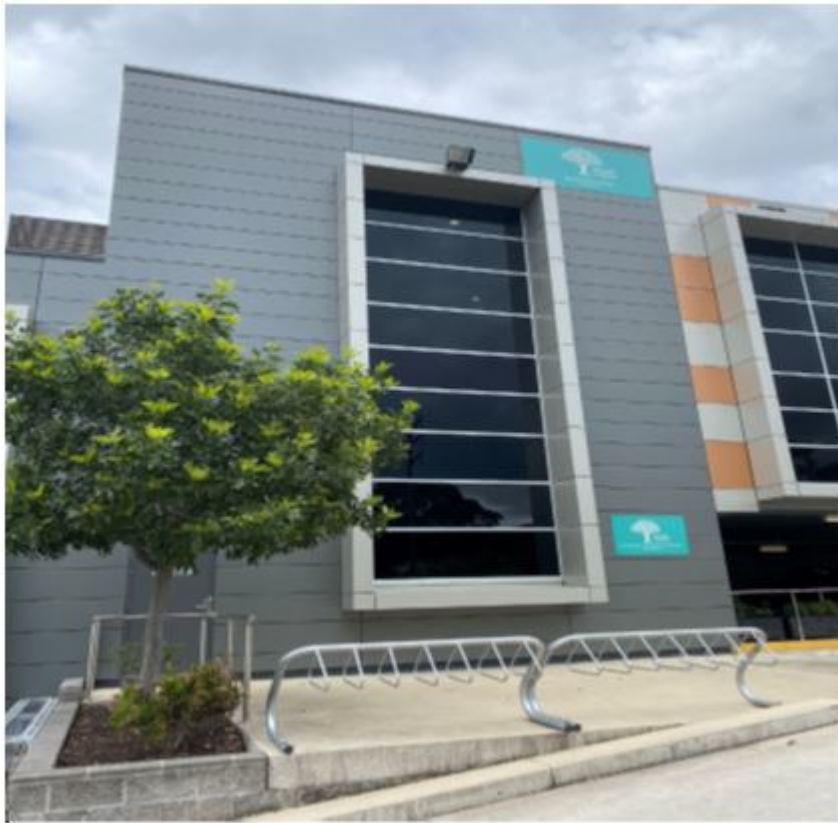
Figure 3 – Photograph of Existing Business Signage – Only About Children Child Care Centre
