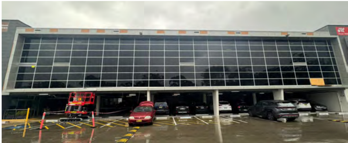
Figure 5 – Photograph of Existing exterior where the Proposed Window Signs will be located.
