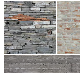
3 Material Reference-Masonry/Off Form Concrete Walls
