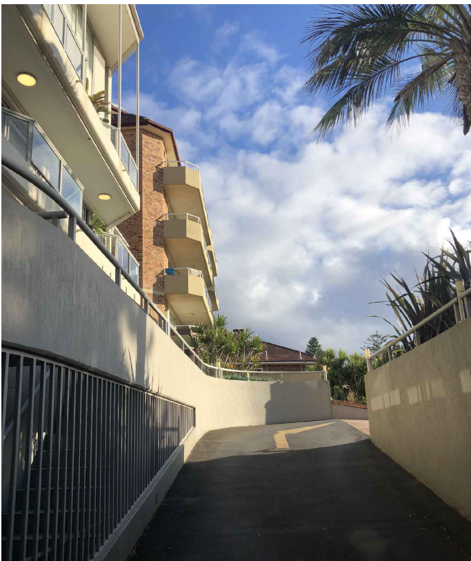
EXIT RAMP FROM BASEMENT TO NORTH STEYNE
