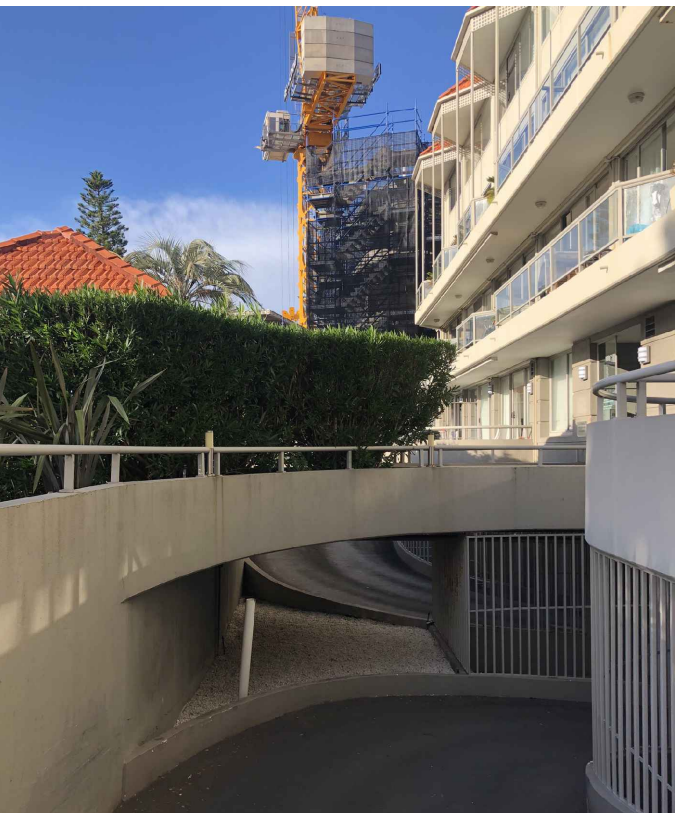
OVERVIEW OF UNDERCOVER SPACE DOWN EXIT RAMP.
