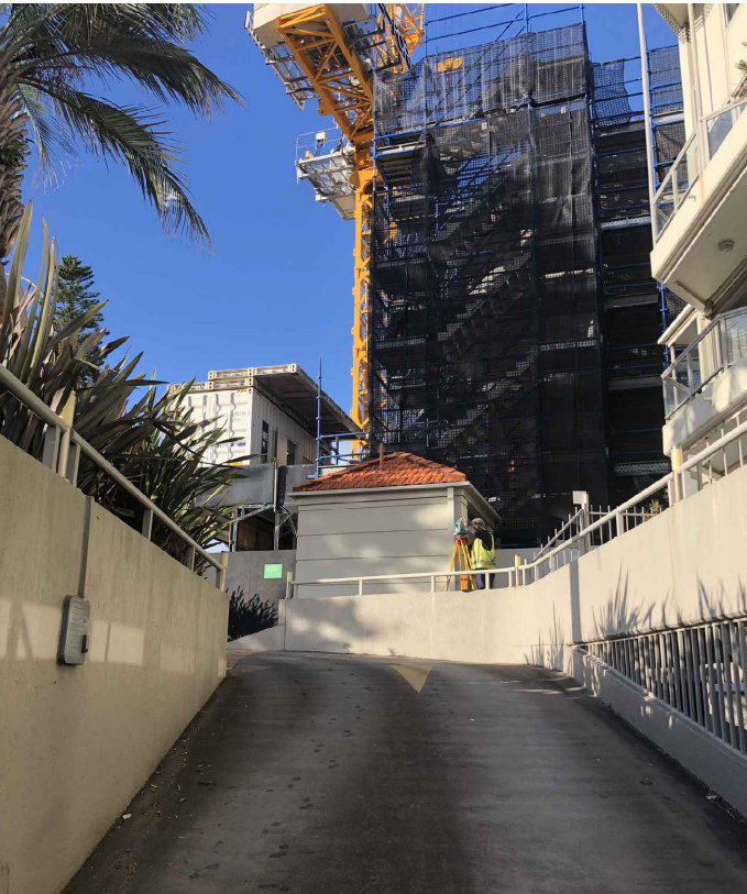
ENTRANCE RAMP FROM BASEMENT TO NORTH STEYNE.
