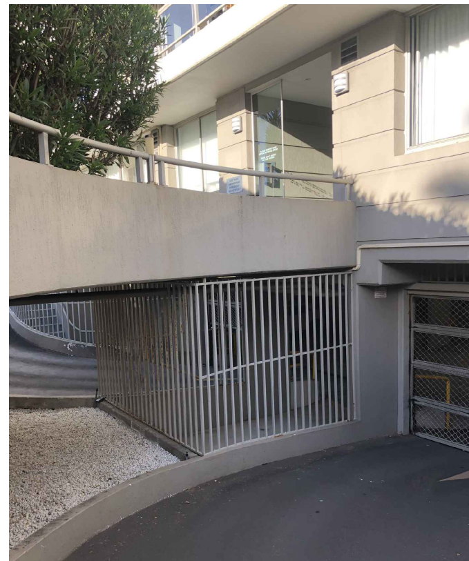
SECURITY FENCING TO STORAGE AND SECURE ROLLER DOORS TO BASEMENT ENTRY.
