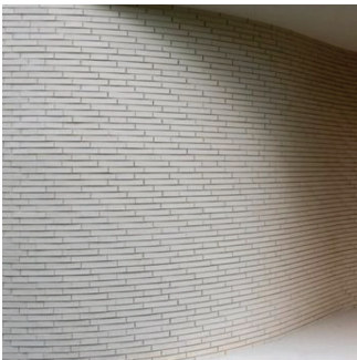
CURVED BRICKWORK WALLS
