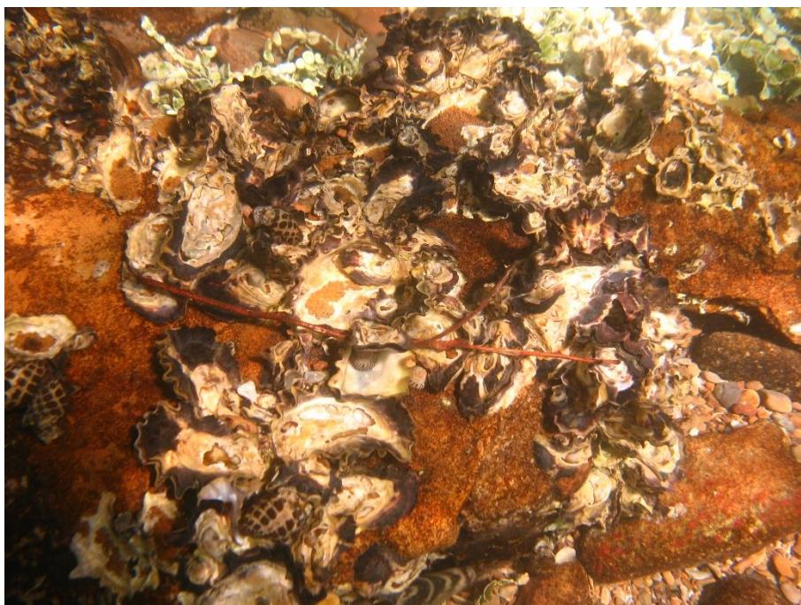
Figure 5. Artificial concrete seawall and small intertidal boulders at the base. Structures were colonised by oysters, various gastropods and turfing algae.
